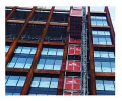
whilst transporting passengers and materials. Depending on the payload a range of geared brake motors can drive the passengers goods hoist cage in the desired direction, up or down. The hoist offers an independent safety function which can bring the cage to a controlled stop in case a combined speed in the downward direction is exceeded.
